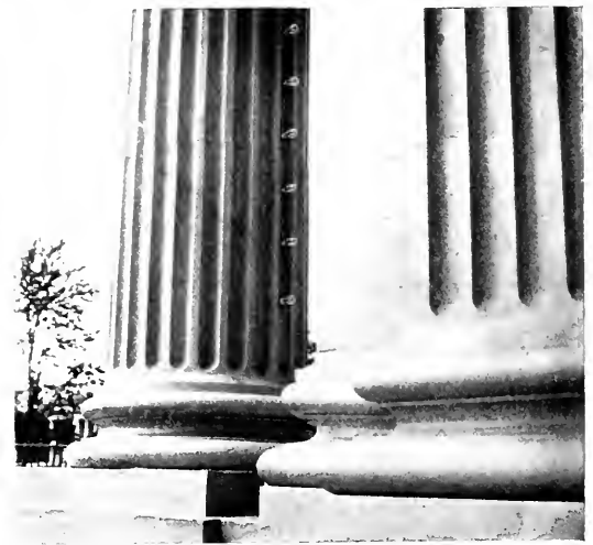
FIG. 7.—EDUCATIONAL BUILDING—LAMPS INSIDE ROW OF COLUMNS.
